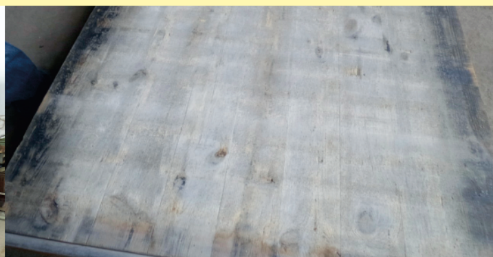
Inspection of the boards
