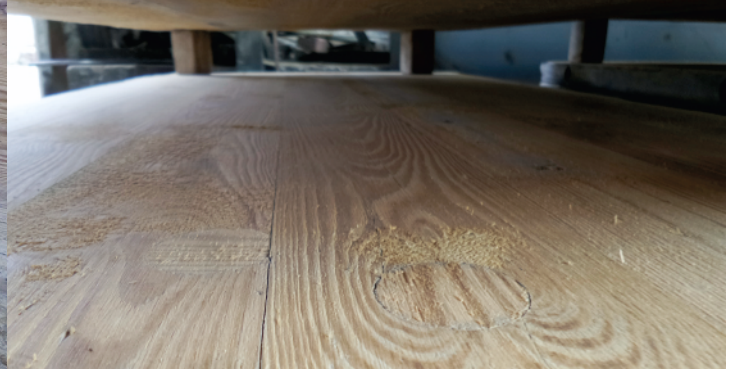
Drilling the defects, plugging the holes
